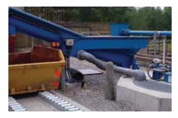
Complete Jeta® grit removal systems can be supplied in steel fabricated tanks. These are ideal for attachment to existing flow channels. Jeta® grit trap sizes up to the 550 size can be supplied in this form.
