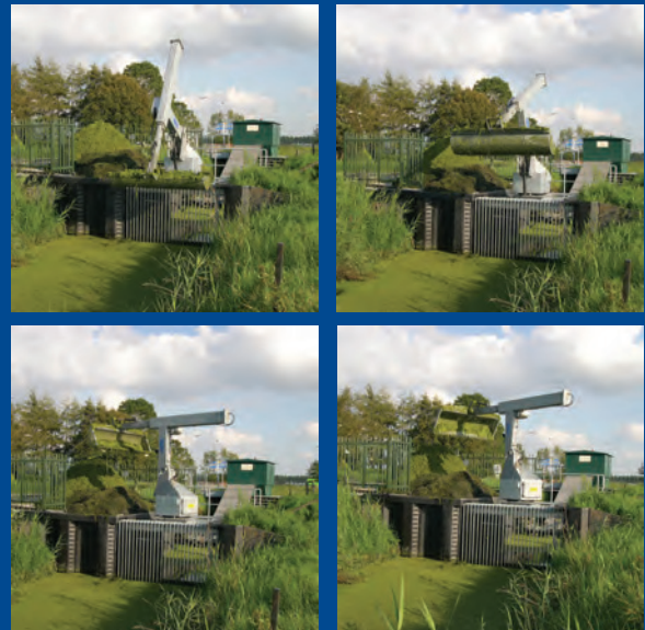
Bosker Bandit automatic trashrake debris being dumped directly into containers for waste treatment or recycling.
